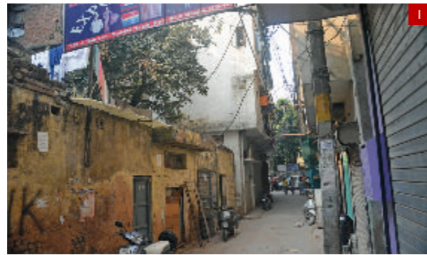
1 Dilapidated structure in Hauz Rani
