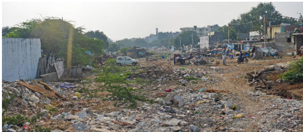
3. Dumping of C&D waste and misuse of ZDP green
