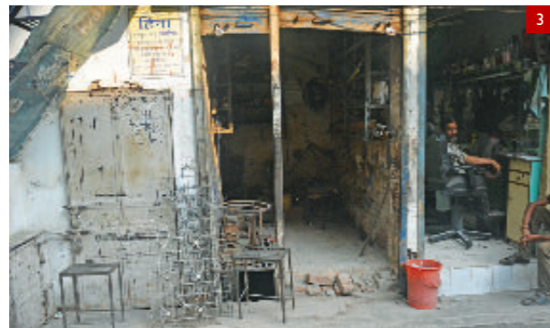
3 Hazardous workshops operating in Hauz Rani
