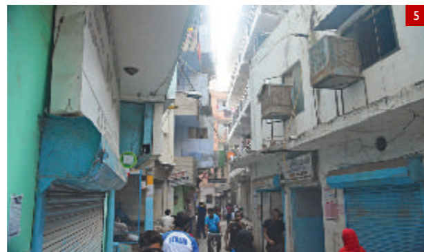
5 Lack of light and ventilation due to building projections and balconies
