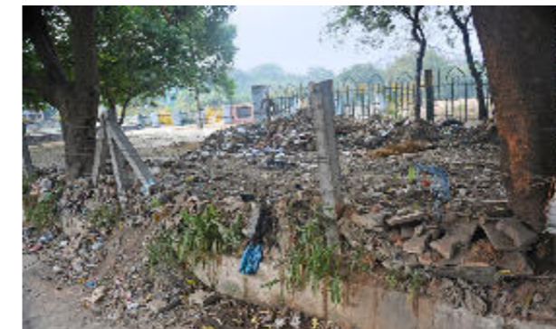
3. Dumping of C&D waste on Pedestrian Walkway
