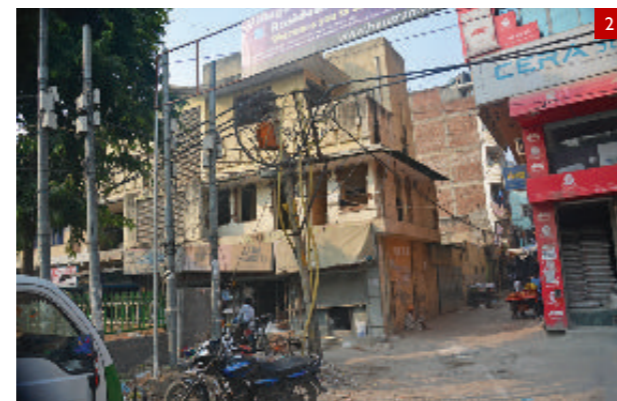
Dilapidated structures and overhanging wiring
